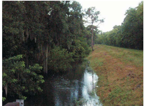
View of the drainage channel south across 118th Ave
