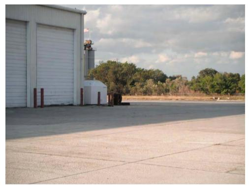
Photograph 5: View of northwest corner of the CCC building - note AST (likely the 3,000 gallon waste oil AST listed in Table 1 of this report).
