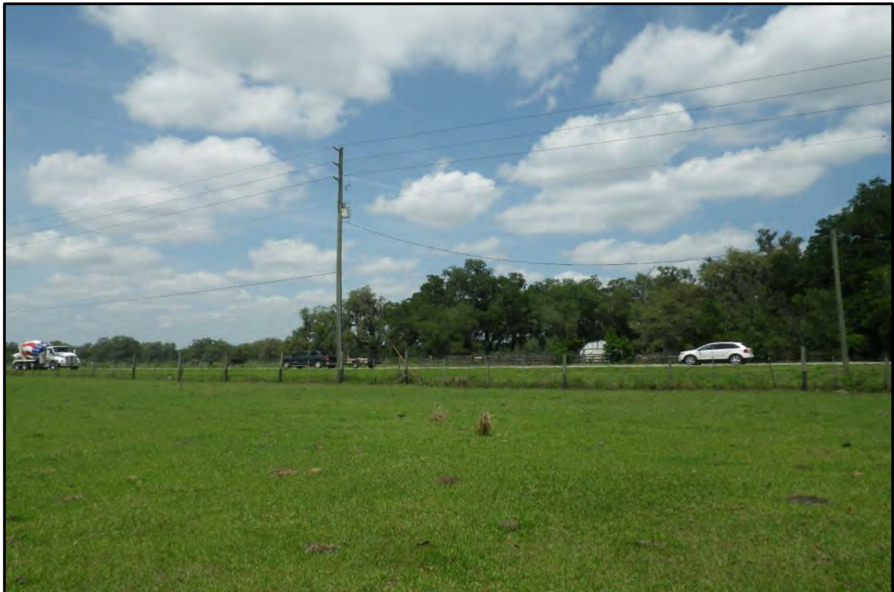
Photograph No. 32 View to the northwest of a pole-mounted transformer located along the northern Subject Property boundary.
