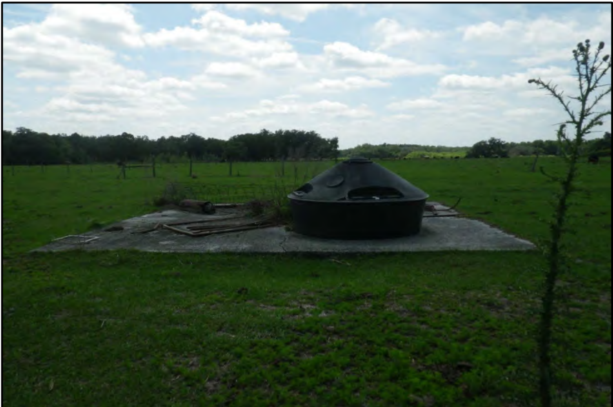
Photograph No. 8 View to the south of a molasses tank, metal pipes, and barbed-wire fence on a concrete slab in the northern portion of the Subject Property.
