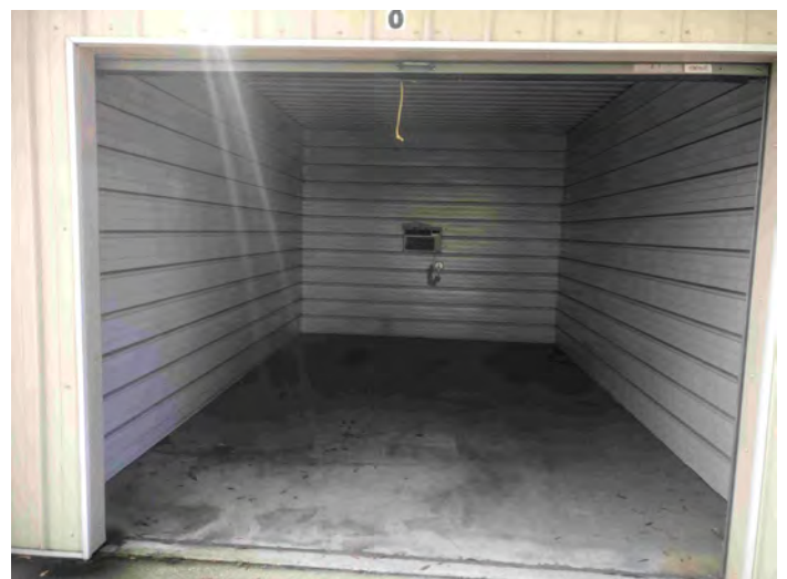
Looking at interior, typical storage unit
