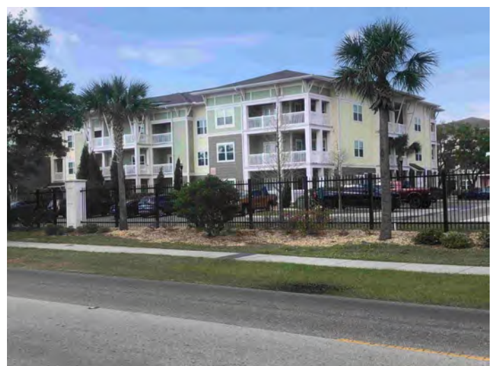
Looking at SW adjoining property
