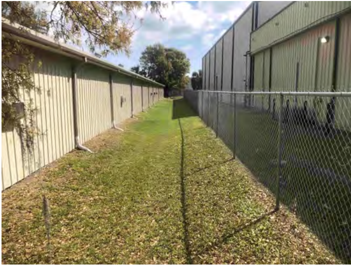
Looking at rear of storage unit Bldg, S property border
