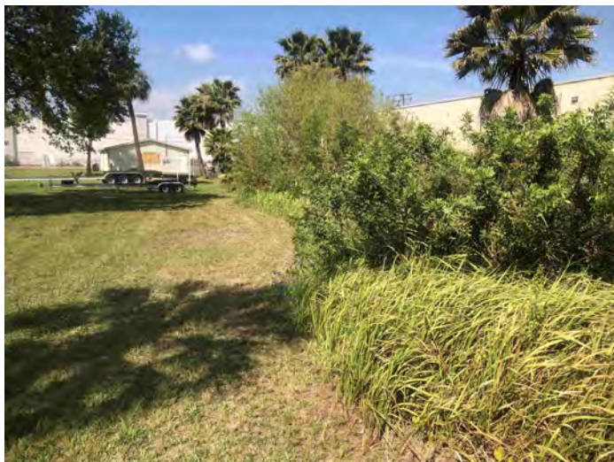
Looking at what appears to be overgrown retention area, N side of Subject
