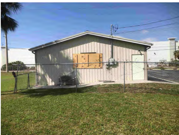
Looking at E side of N structure on property line
