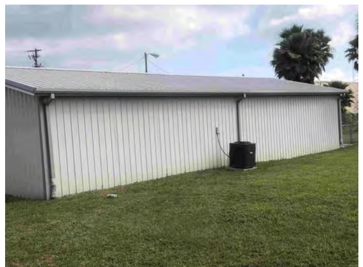
Looking at S side, N building
