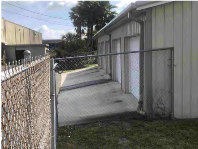
Looking at N side of N building, opens onto adjoining property to the N
