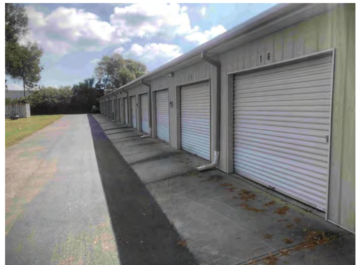
Looking at storage units
